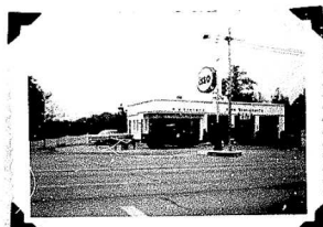
M.W. Roberts "Esso" Service Station S.E. Corner Stevenson Lane & York Road.
