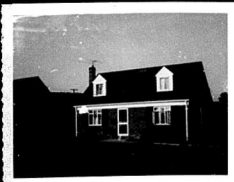
5th house south of Warren Road, East side of Greenleaf Rd.
