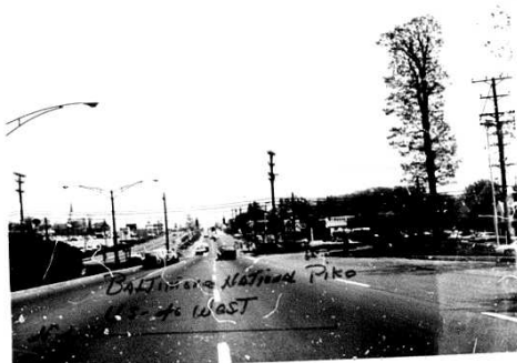
BALTIMORE NATIONAL PIKE U. S. 40 WEST CATONSVILLE, MARYLAND
