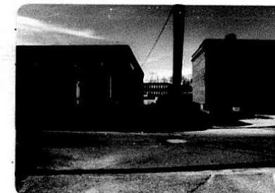
Pikesville Sub-station Photographs
