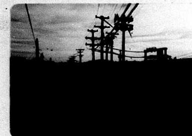
Halethorpe Sub-station Photographs
