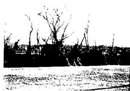
M. HARBOR TUNNEL ROAD LOOKING SOUTHWEST FROM KRONHEIM
