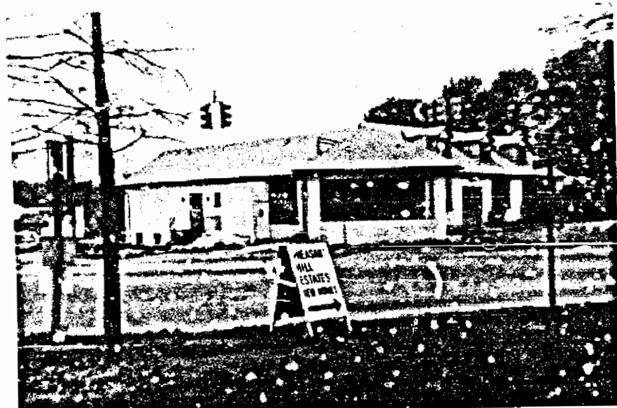
1)- Taken Saturday morning, April 26, 1980. The subject property seen from diagonally opposite (building assoc. parking lot)
