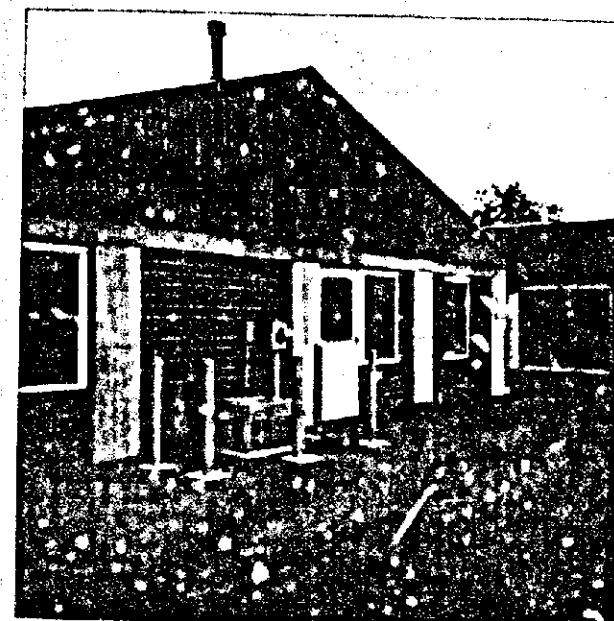
Resident Manager's Apartment and Office at end of Bldg #1
