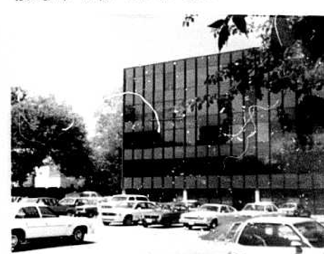
T. PARKING LOT AND REAR OF CHESAPEAKE BUILDING ON S 1/2 OF CHESAPEAKE AVE., NW OF SITE
