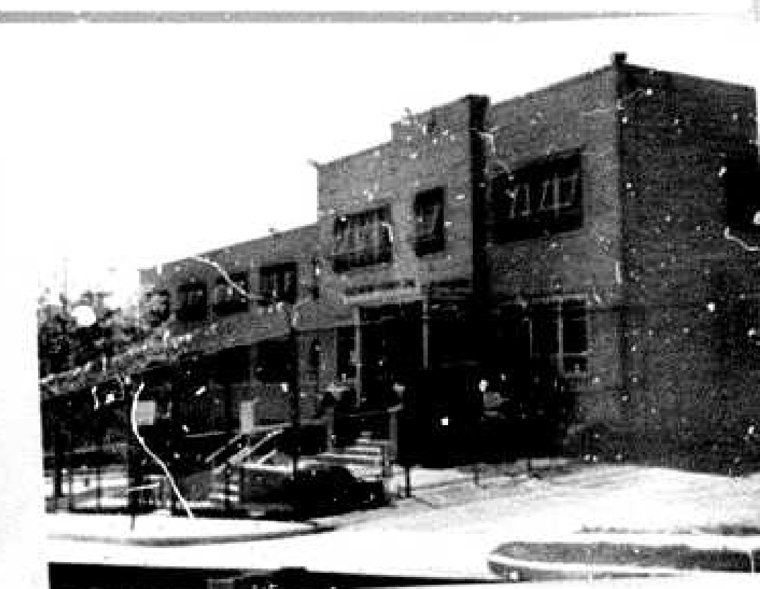
W. FRONT OF WORK RELEASE CENTER SE OF SITE FROM NEW BOSLEY
