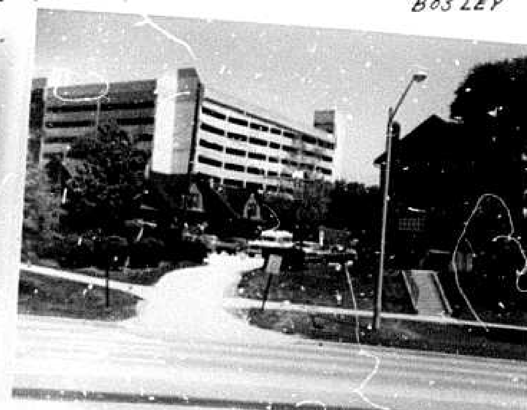
K. COUNTY OFFICES ON NE 1/2 OF NEW BOSLEY OPPOSITE SITE BETWEEN TWO PROPOSED ENTRANCE SITES
