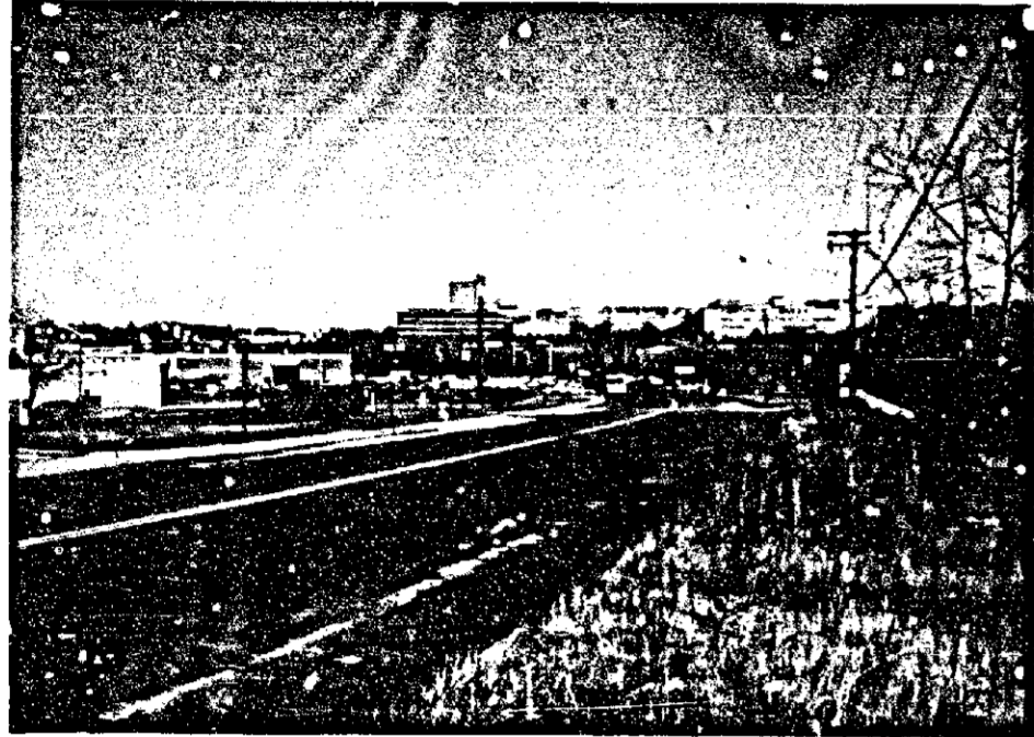
A. EX. FRONTAGE - LOOKING EASTERLY ALONG WHITEHEAD CT.
