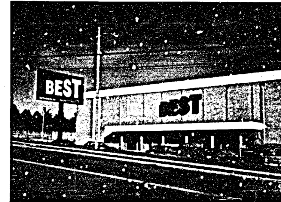
E. VIEW OF EXISTING BEST PRODUCTS BLDG. & FREE STANDING SIGN ON WHITEHEAD ROAD
