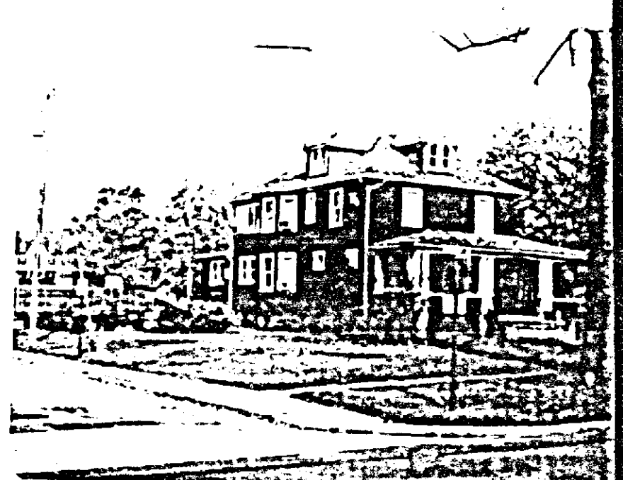
C. Looking N/Ely AT THE SEIPP PROPERTY 408 ALLEGHENY AVE.
