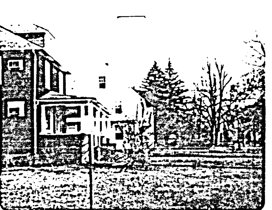
D. Looking E/ly past Seipp pole, and poles, to the E on N/S of Allegheny
