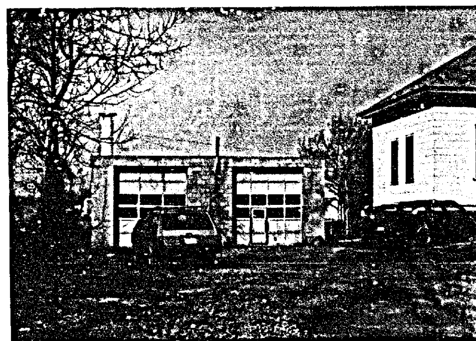
Block Garage - Viewed from Hollins Ferry Road
