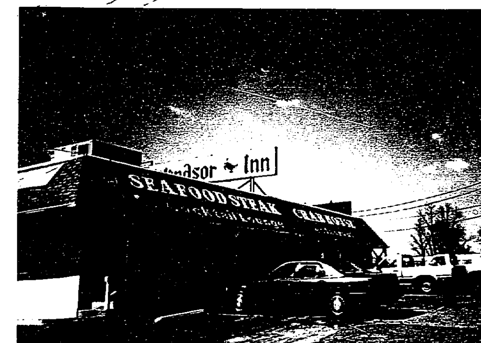
WINDSOR INN, WINDSOR MILL ROAD ELEVATION
