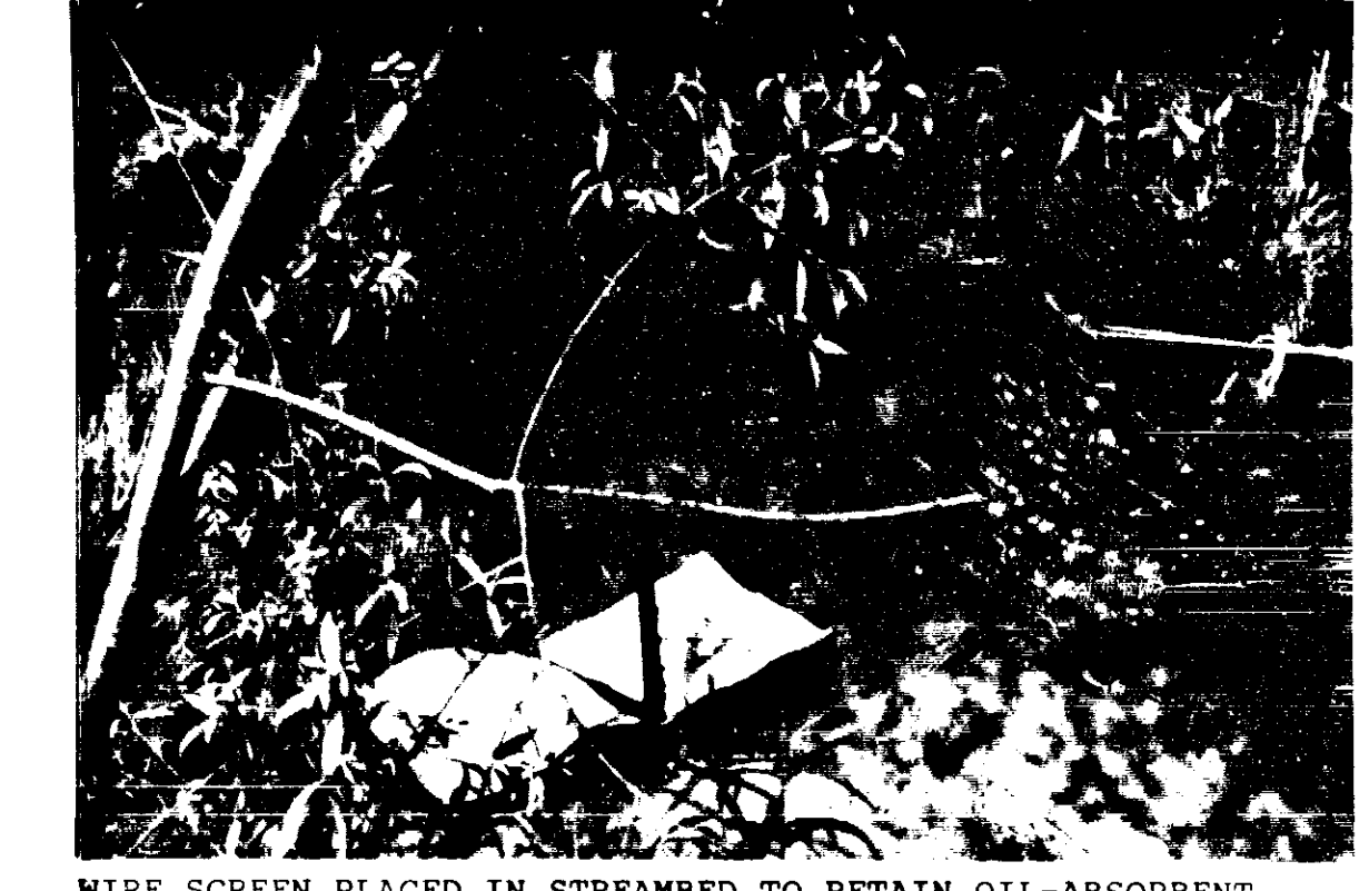
WIRE SCREEN PLACED IN STREAMBED TO RETAIN OIL-ABSORBENT MATERIAL AT THE GSEI DRIVEWAY.
