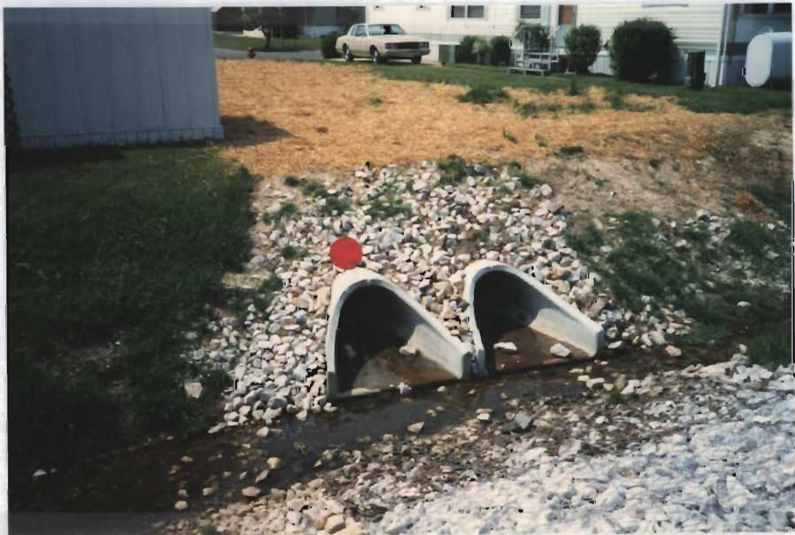
RED DOT: New drain along with new end section to original drain.
