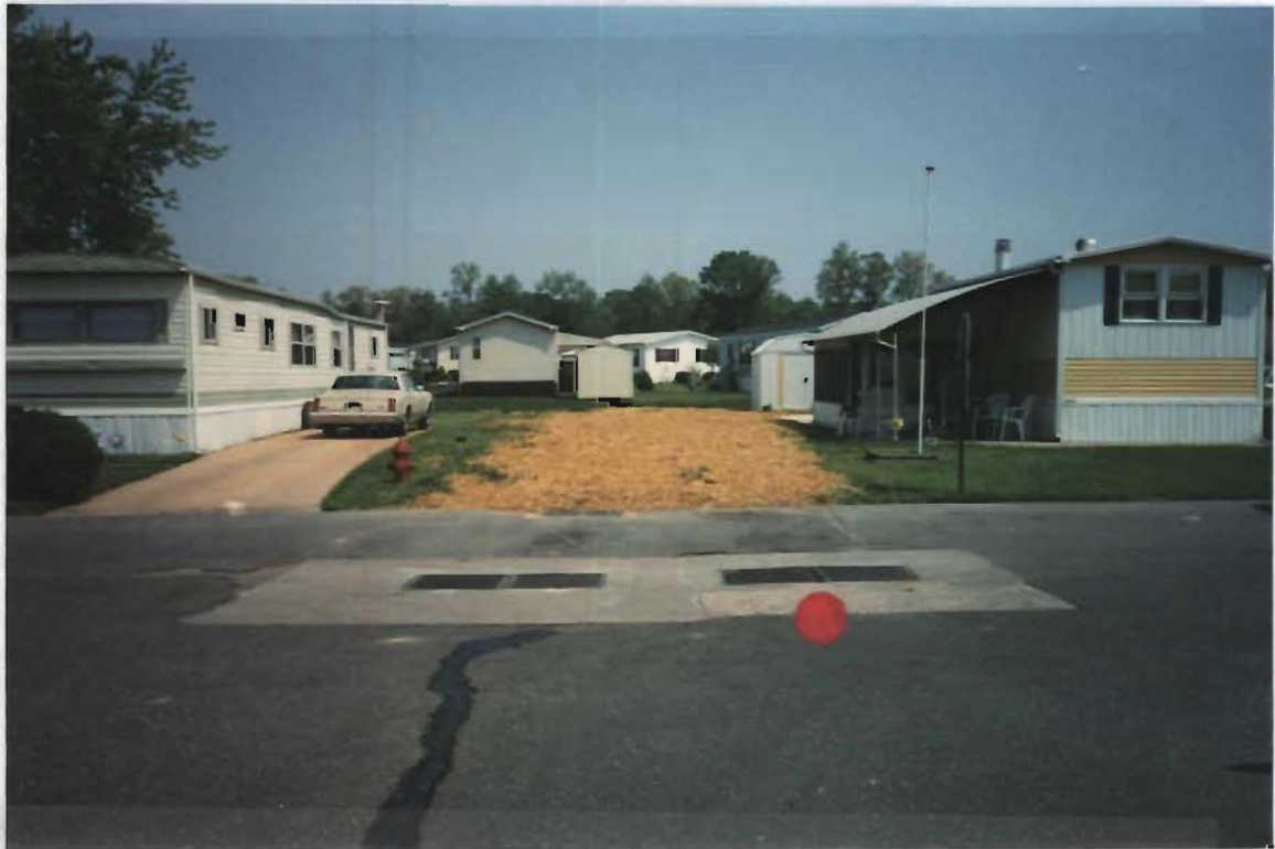
RED DOT: Additional Drain Installed.
