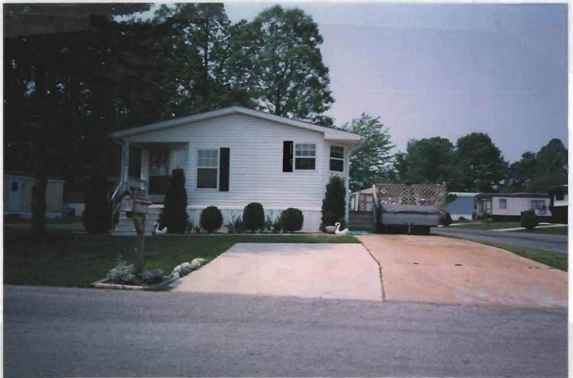
New double wide home replacing previous older single wide home on Wheelhouse Road.
