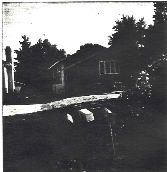
House being built across St. from this property BLDG Lot
