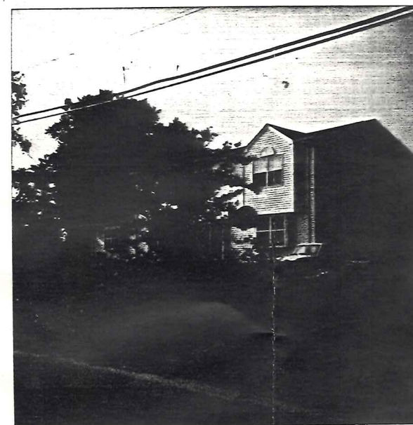
Ex. House on West side (Adjacent Lot)
