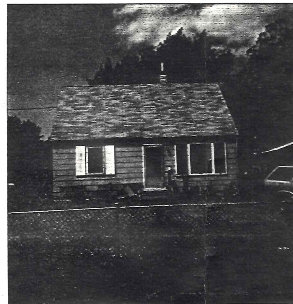
Old House Razed Prop. site
