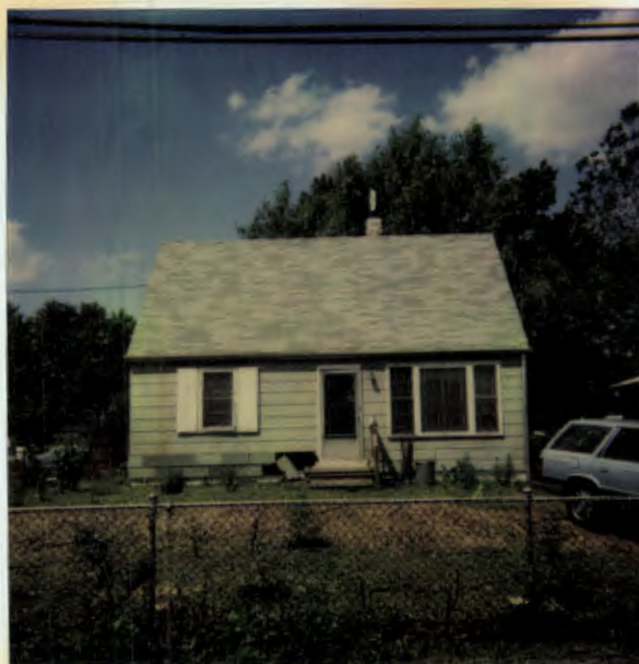
Old House = Razed PROP. site
