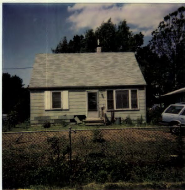
old House RAZED Prop. site
