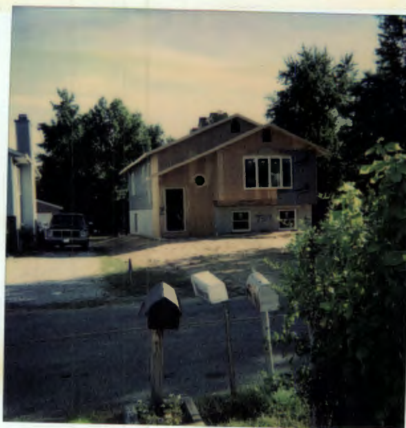
House being built across ST. from this property BLDG 12
