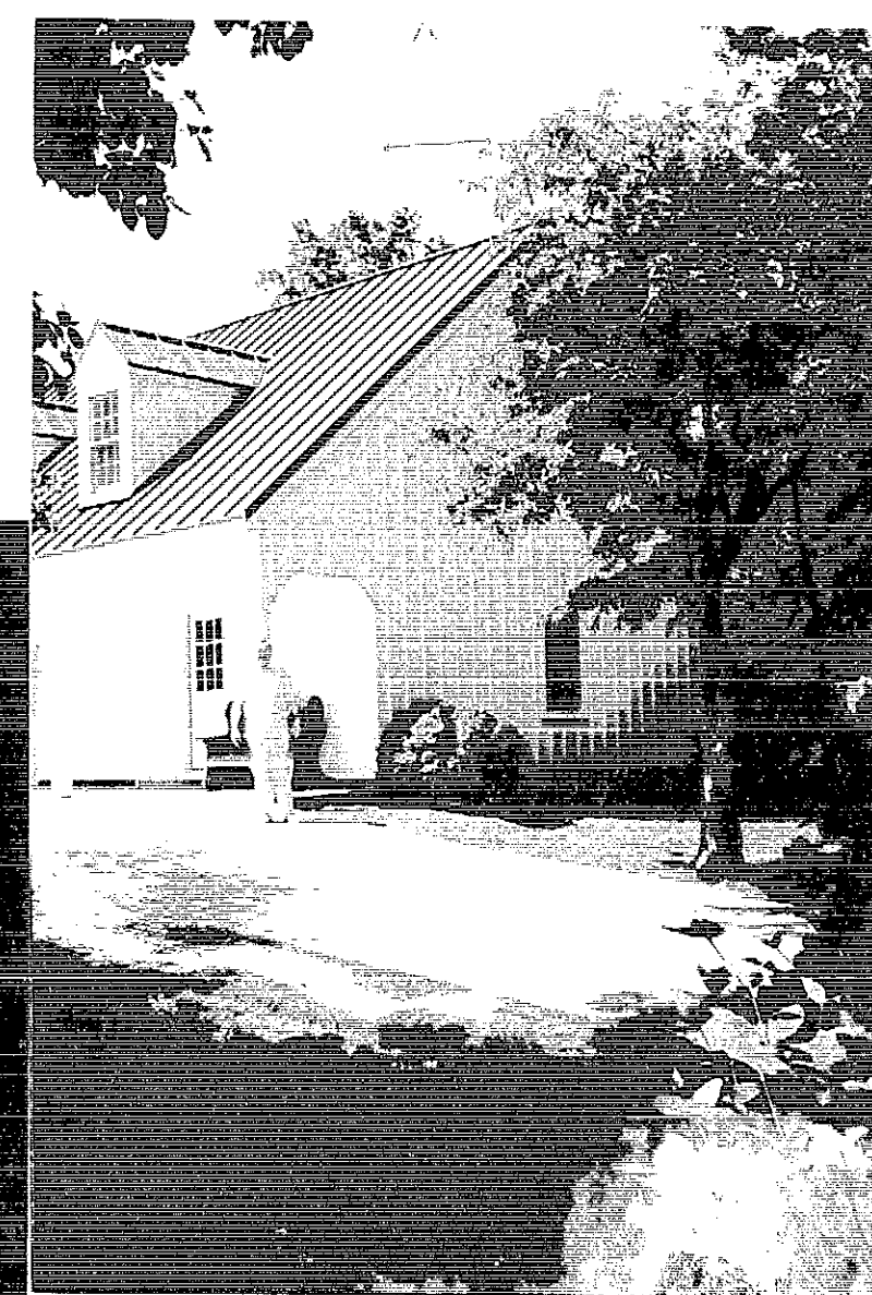
I. North end of Ward Garage, looking southwest
