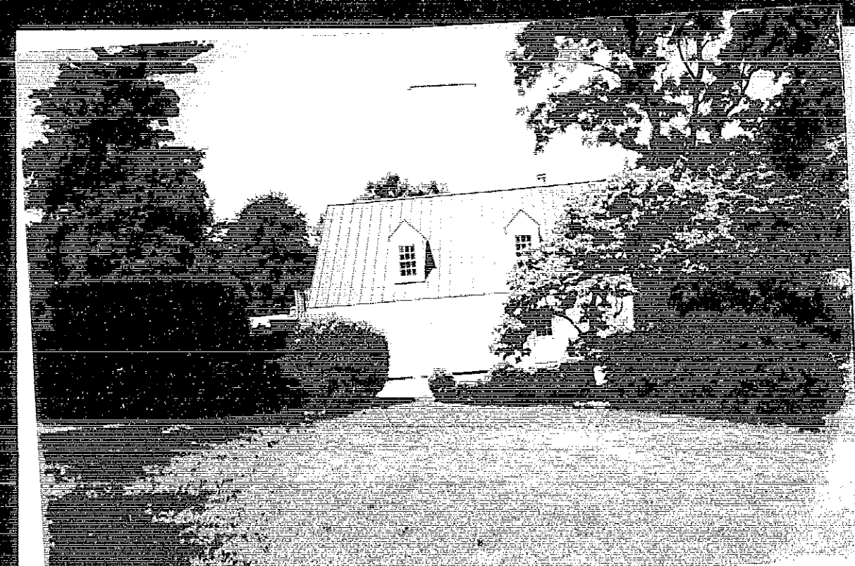
G. Ward Garage, Wine Cellar and Storage Building looking west
