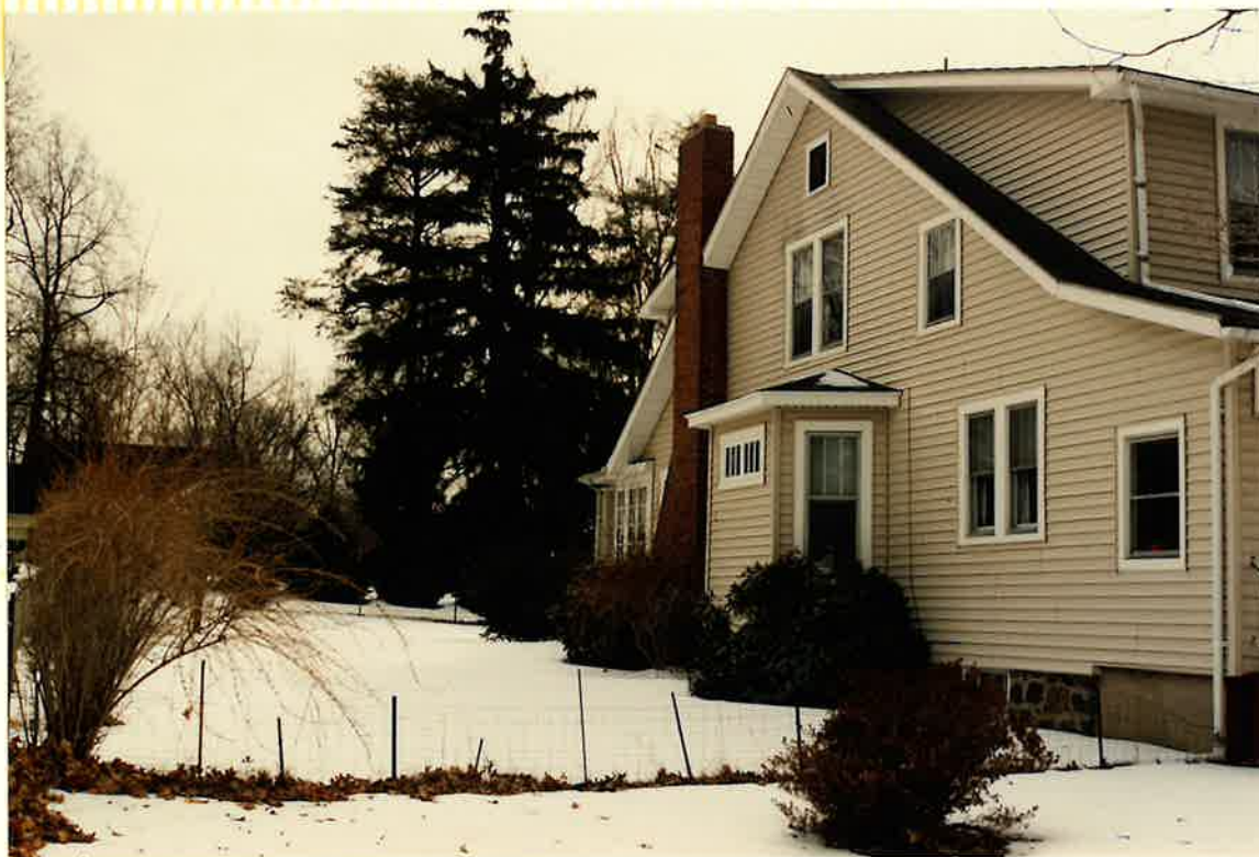
LEFT SIDE OF HOUSE FROM THE BACK
