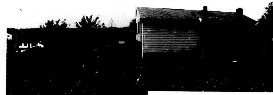
Rear of House
