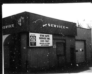
F. 1024 York Rd - Service Garage. Star Auto
