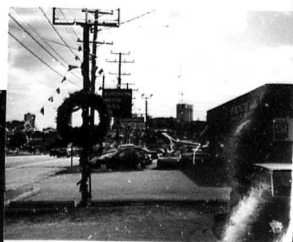
H. Looking South from adjacent property
