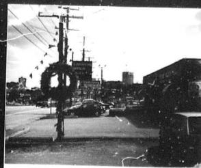
C. Front view of 1020 and 1024 looking South
