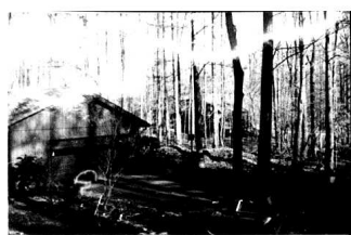
J. Looking southwest at garage on west end of 2319 Velvet Ridge Drive
