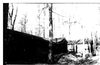
I. Looking southwest at 2319 Velvet Ridge Drive
