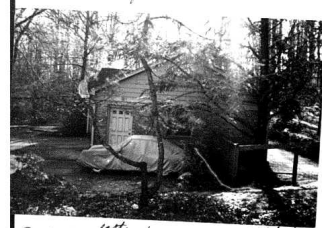
E. Looking west at 2317 from 2319 Velvet Ridge Drive
