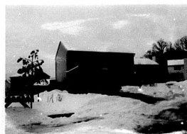
Photo 4 View of subject property from Topsfield Drive.
