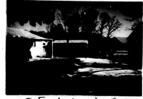
S.E. elevation. Item # 348
