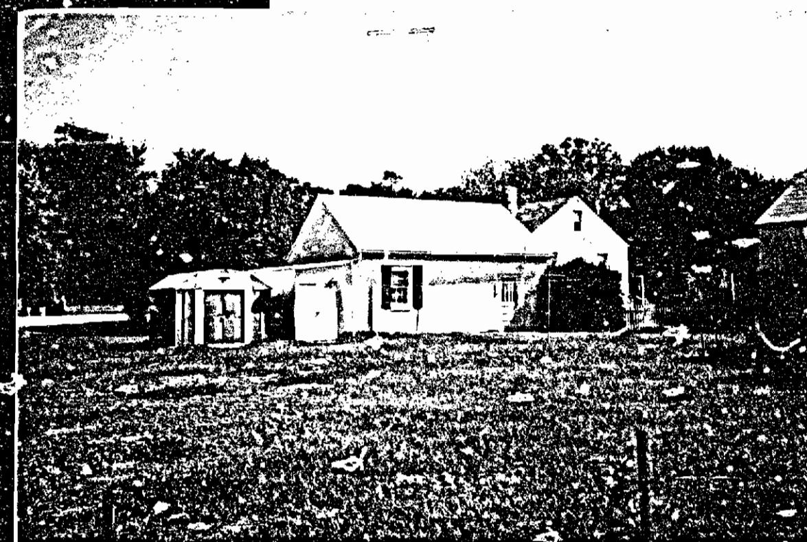
W. Rear of Tripp from Avey, Garage, Corner of House on right
