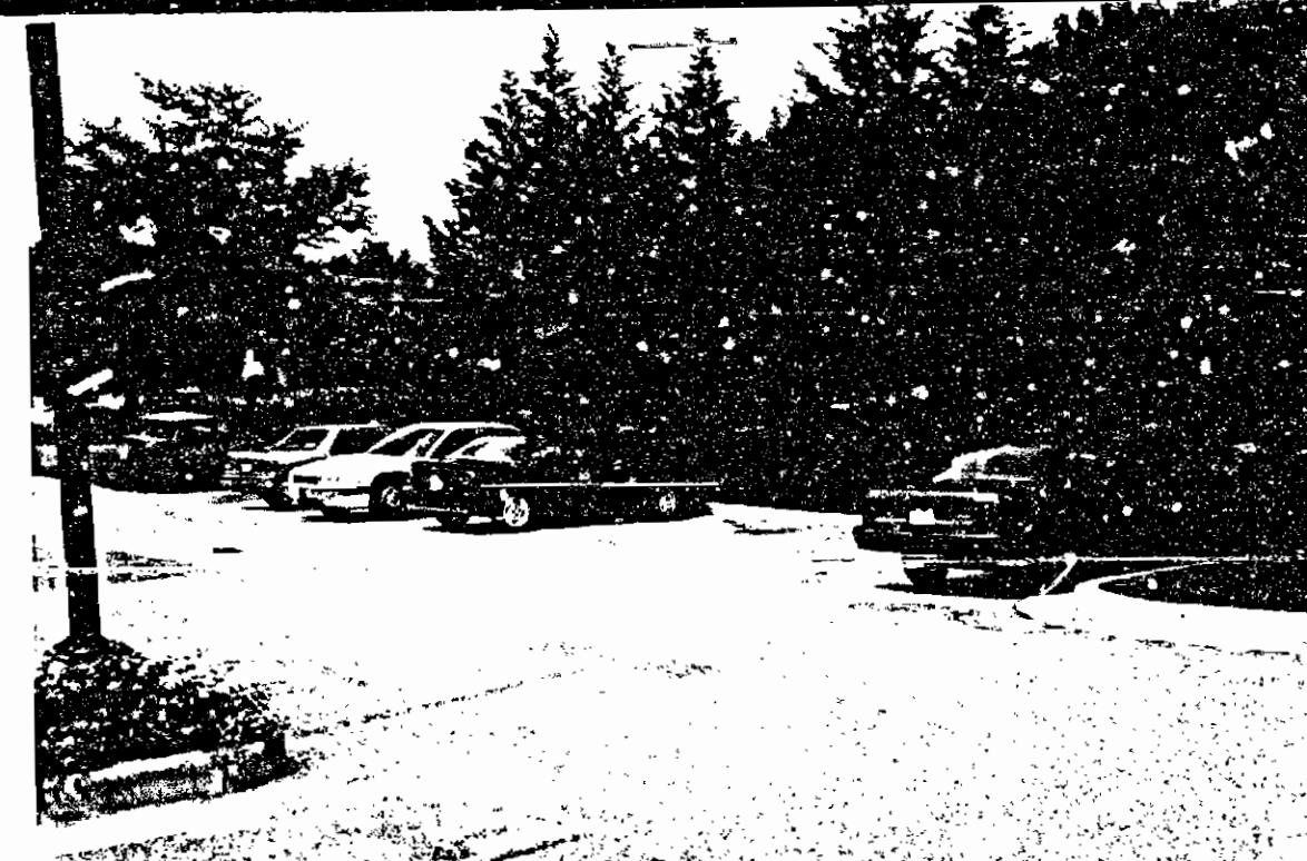
D. Present Rear of Harvest Lot - Note height and density of landscaping - 8' wide strip
