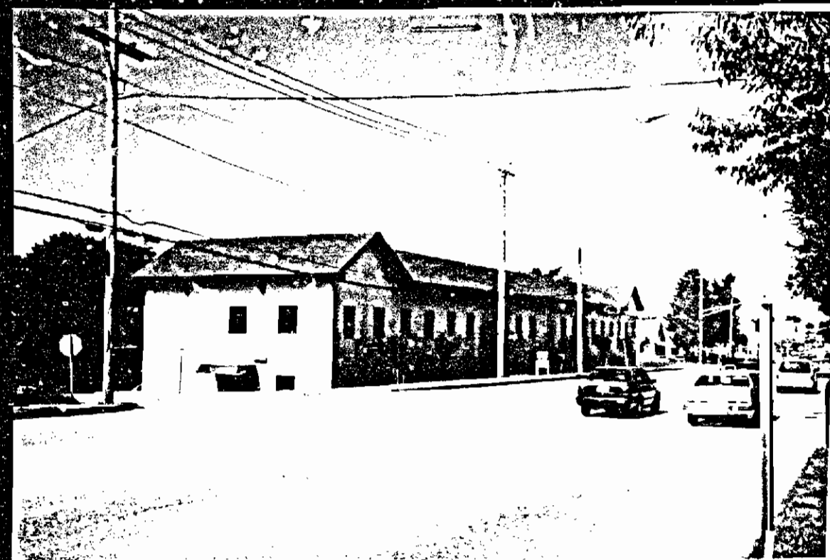
K. Building on W/S of York Rd., N of Harwest
