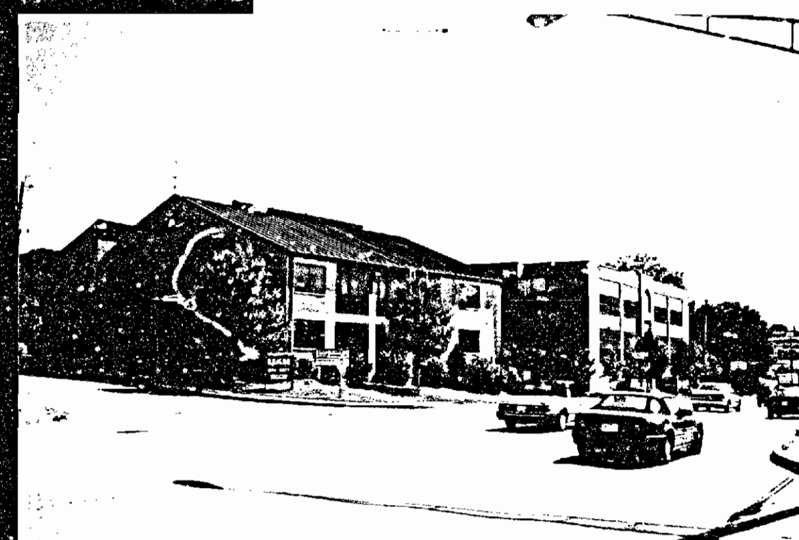
O. Former Maryland Communications Bldg. at SE/C of York Rd. and Tallott Ave., on E/S of York, One Property to S of Harwest
