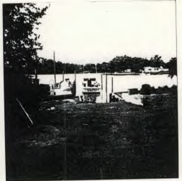
EXISTING CONDITIONS 7831 DENTON ROAD
