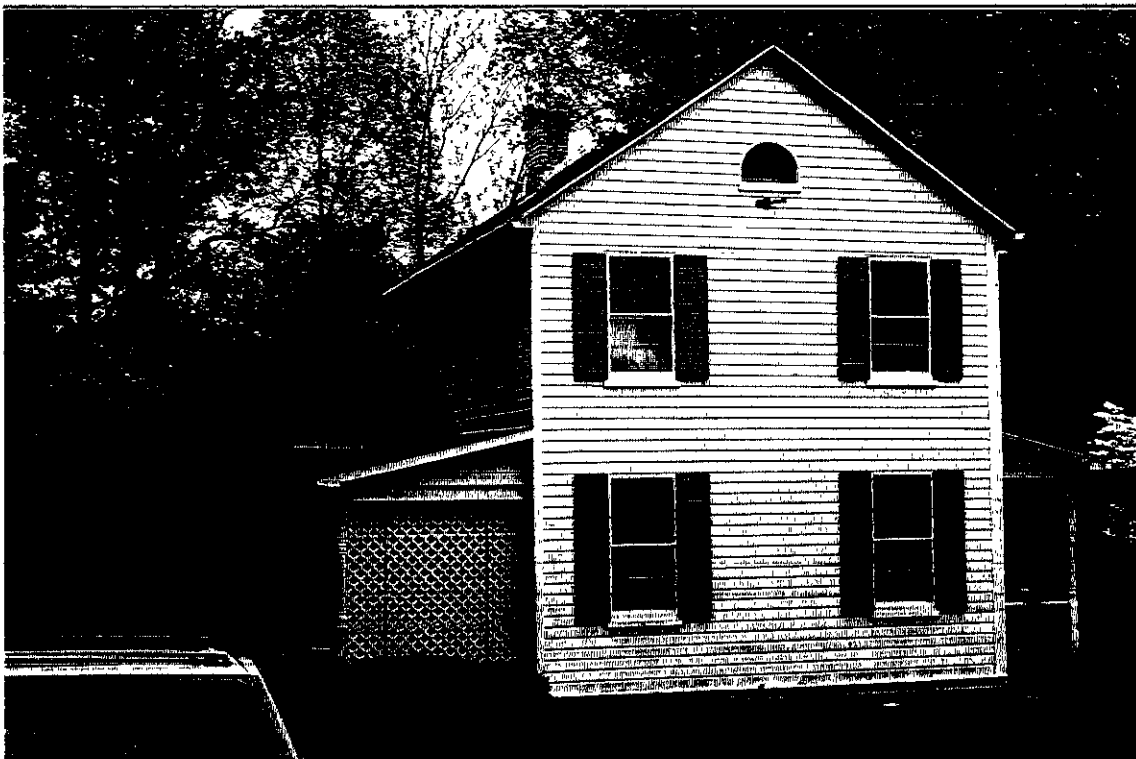
VIEW: WEST VIEW TOWARDS HOUSE
