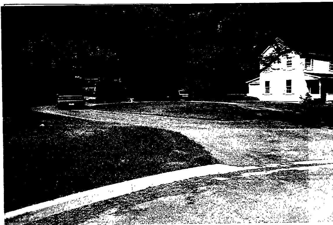
VIEW: SOUTHWEST VIEW TOWARD PROPOSED ADDITION BUILDING AREA
