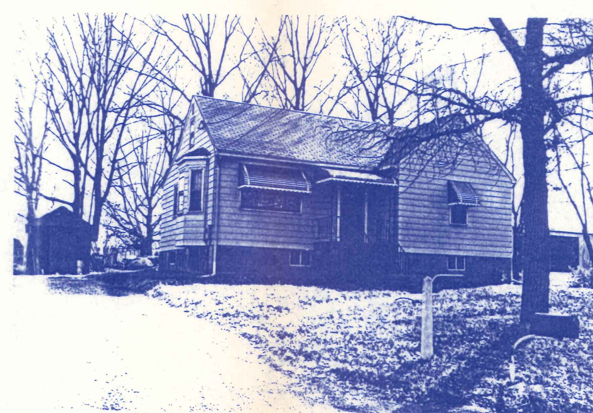
PROPERTY ON RIGHT SIDE OF SITE
