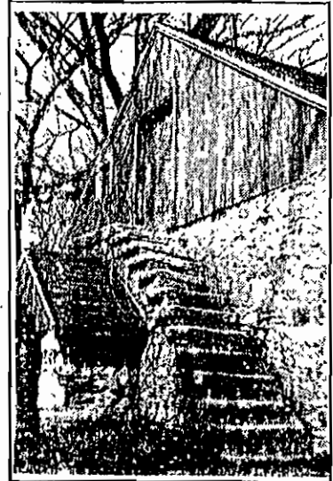
These stone steps lead to the garret above the fieldstone wagon shed.
