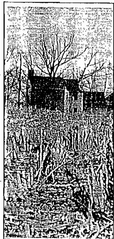
The bachelor quarters are in rack and ruin, sorely in need of major overhaul.
