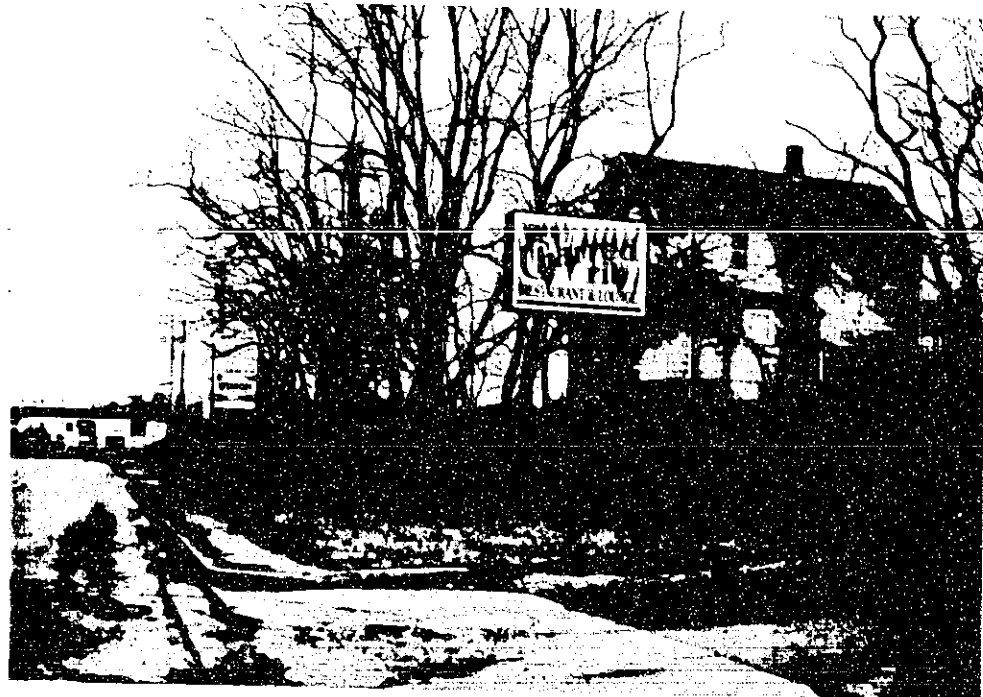
W. AYLESBURY ROAD VIEW LOOKING NORTH
