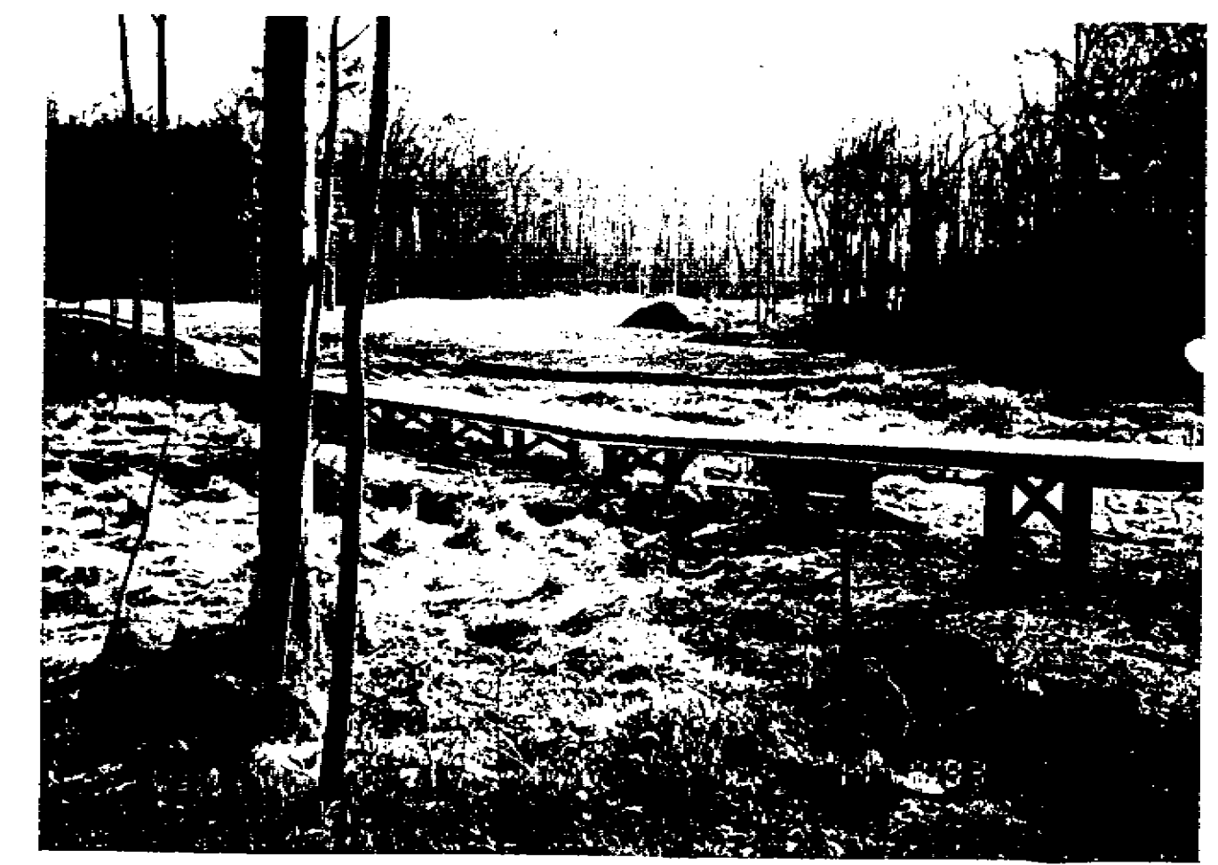
WOOD POST BEAM & PLANK BRIDGE OVER WETLANDS
