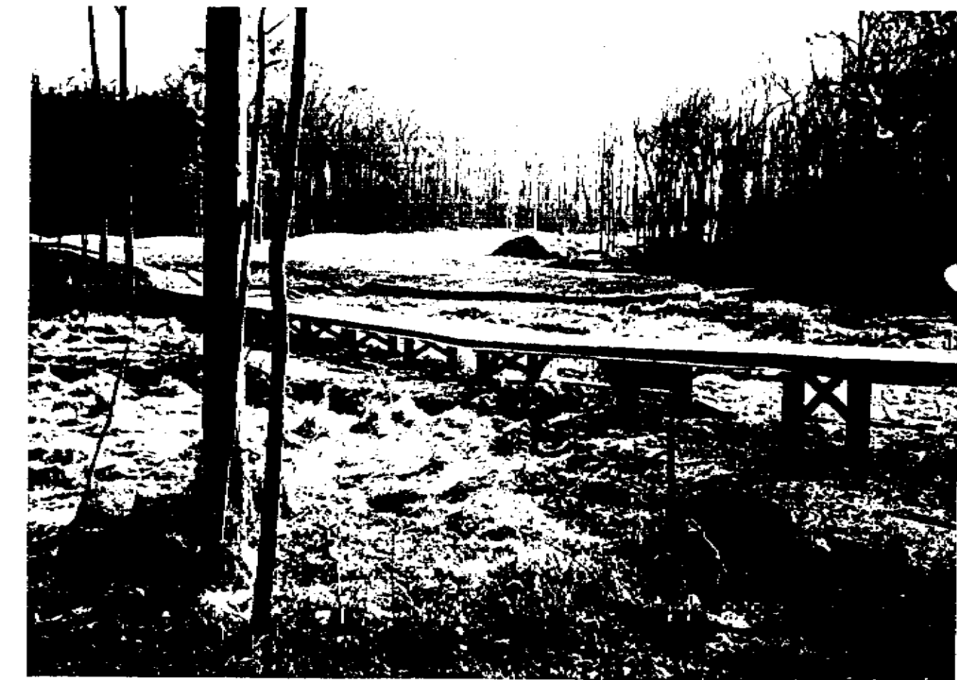
WOOD POST BEAM & PLANK BRIDGE OVER WETLANDS
