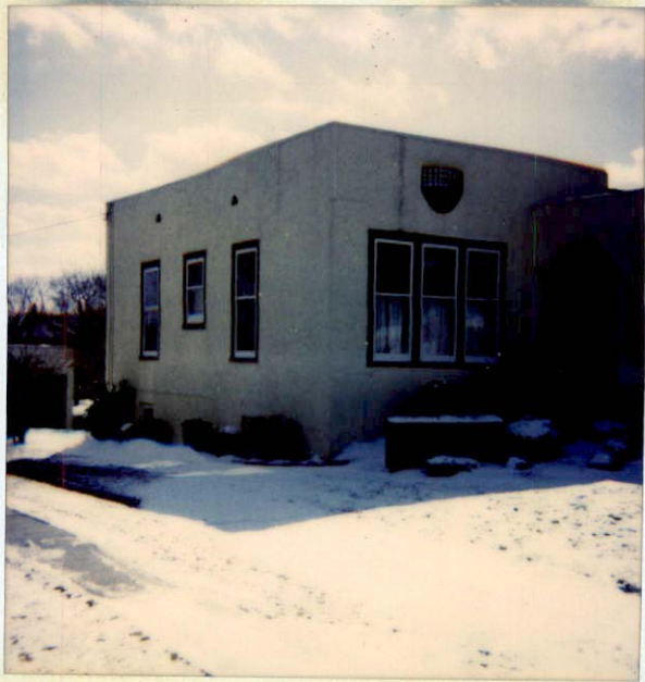
South view side OF House
