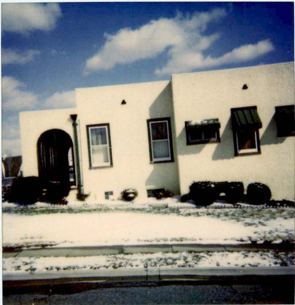
NORTH view side OF House
