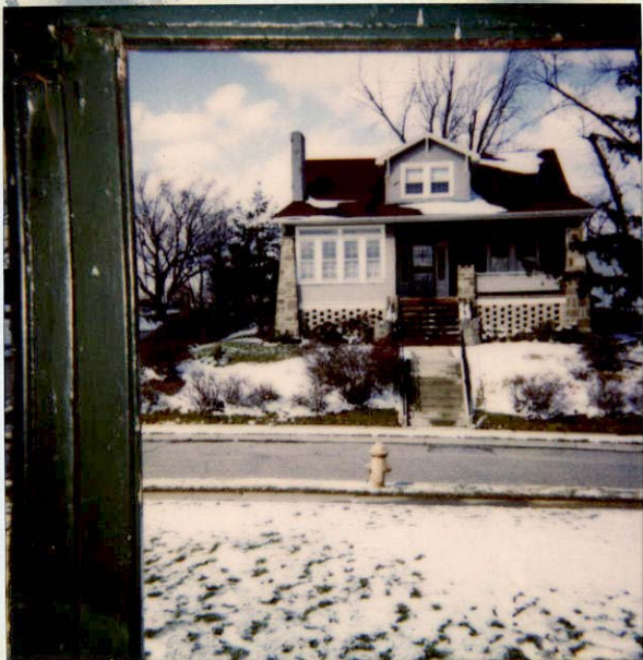
VIEW FROM Front Porch view - EAST
