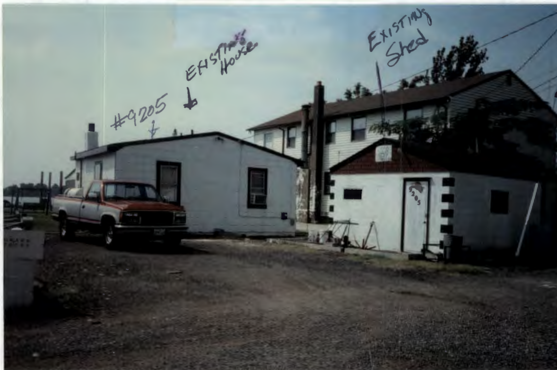
FROM ROAD FRONT, WEST SIDE OF HOUSE
