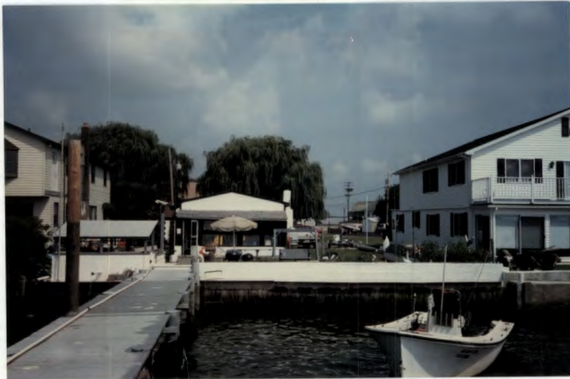
VIEW OF NORTH SIDE ADJENT HOUSE FROM THE EAST
