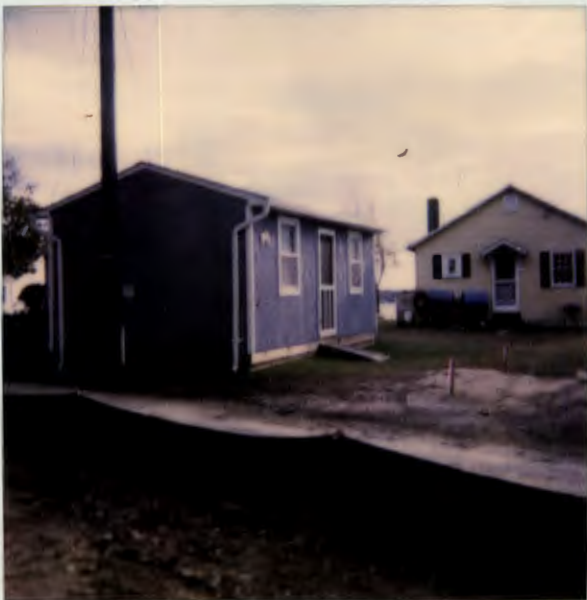
ROAD SIDE (REAR) LOOKING SOUTH
