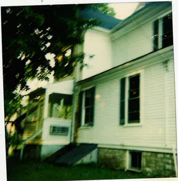
639 main Street Rear Entrance (Right)
