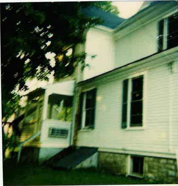
639 main Street Rear Entrance (Right)
