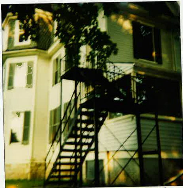
639 main Street Rear Entrance (Left)
