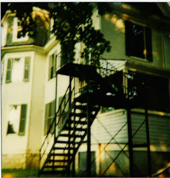
639 main Street Rear Entrance (Left)
