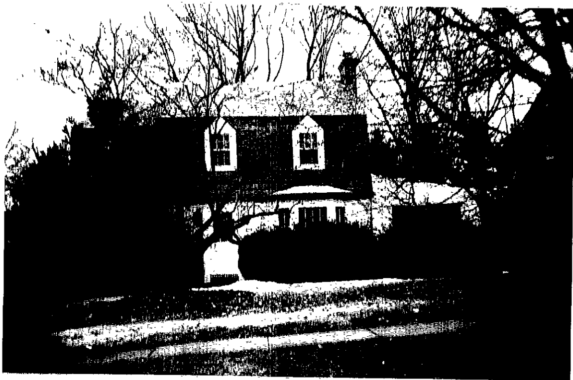
Side addition at 411 Alabama Rd. 290
