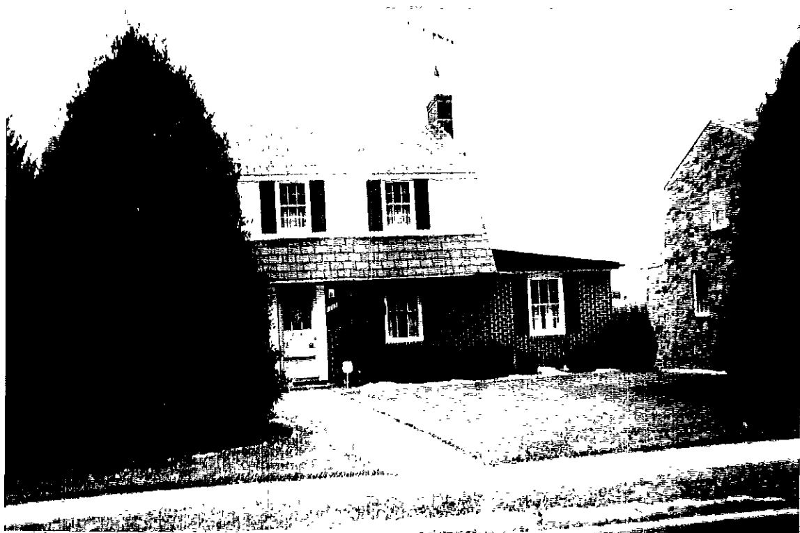
Side addition at 433 Alabama Rd.
