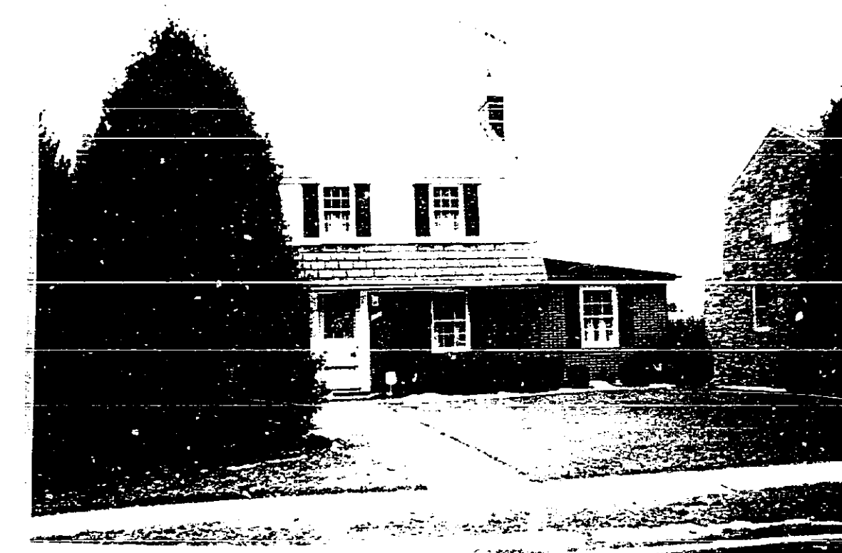
Side addition at 433 Alabama Rd.
