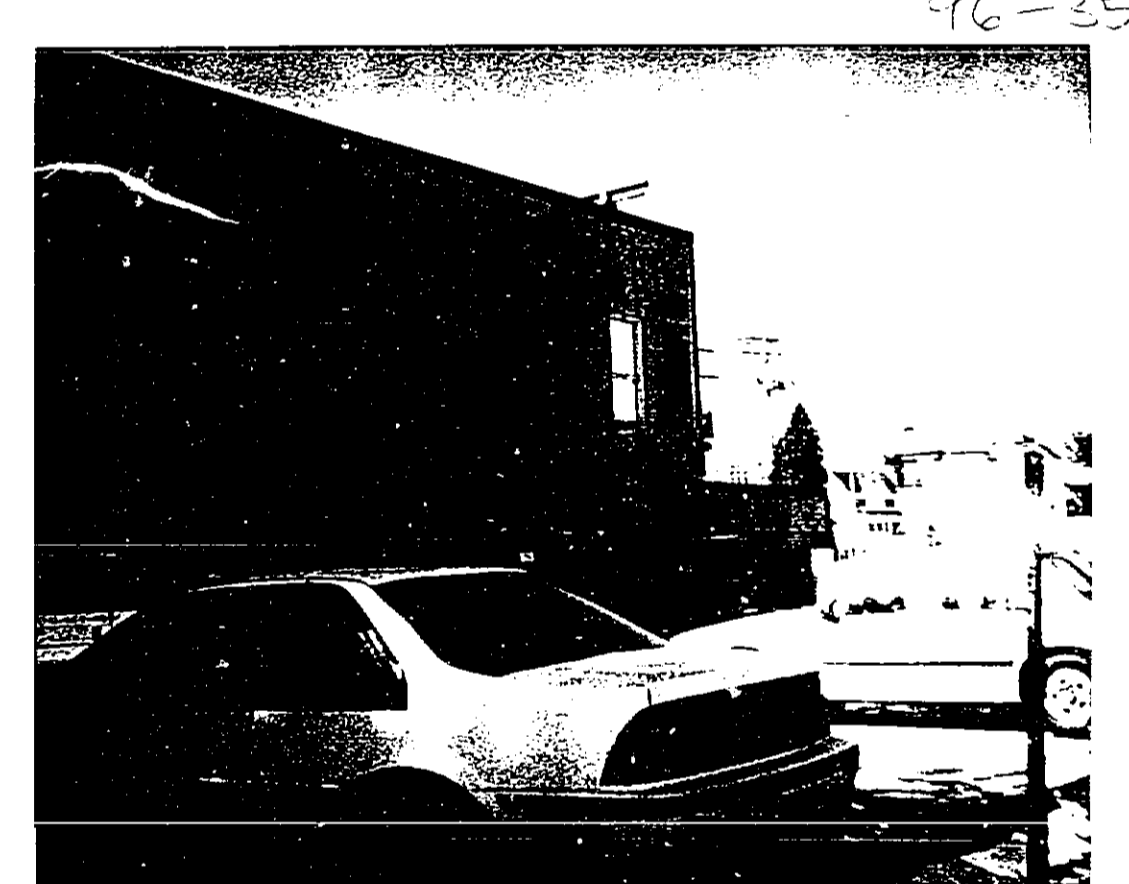
REAR OF BUILDING/PARKING AREA
