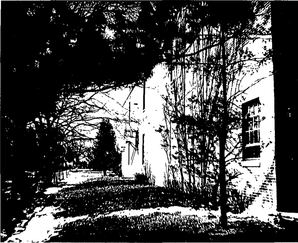
EAST SIDE OF BUILDING
