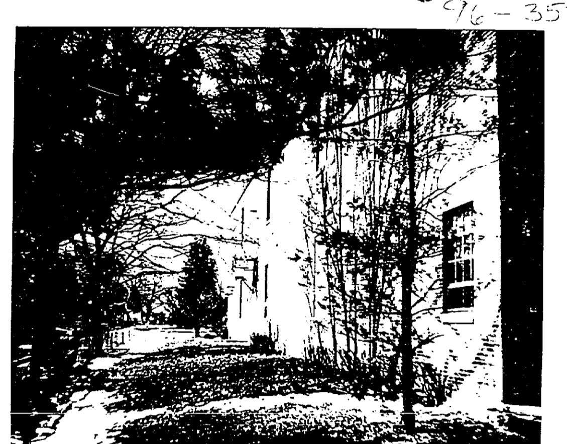
EAST SIDE OF BUILDING
