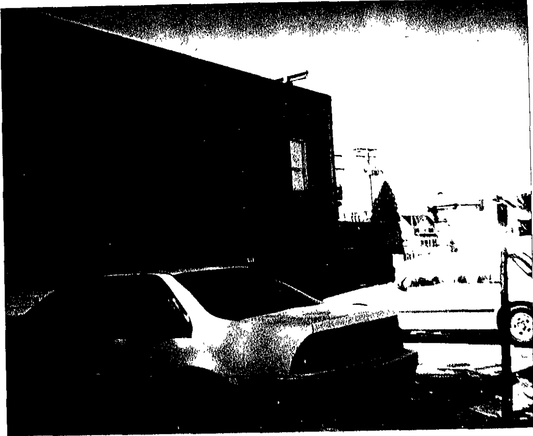
REAR OF BUILDING / PARKING AREA
