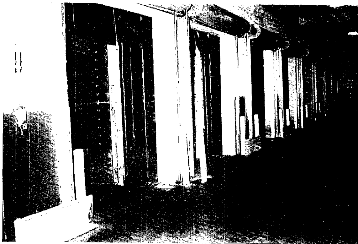
LAST #1 TRUCK BAYS #13 TO 20
