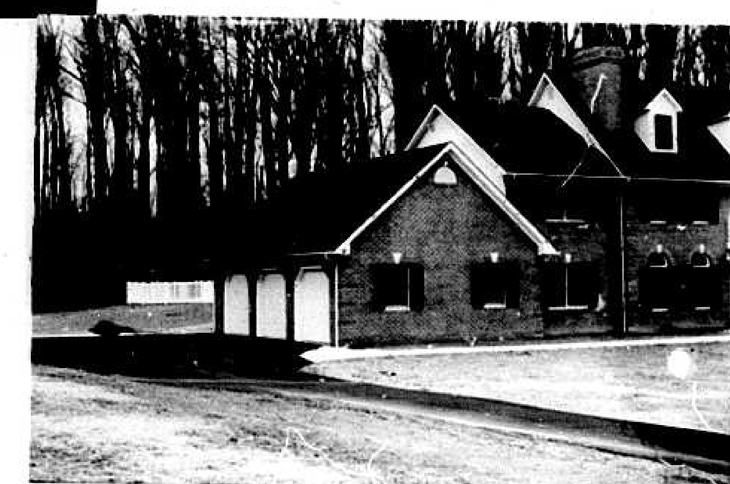
F. North end of Parker Home - 3 Garages.
