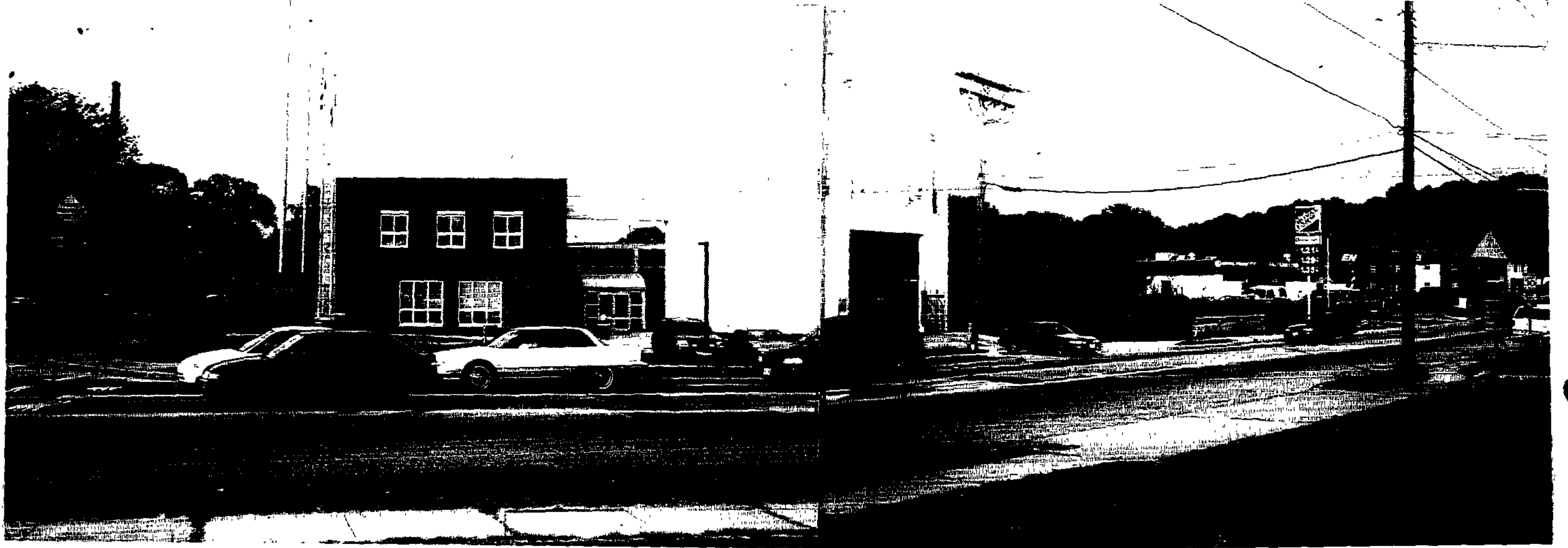
D. Looking NE across Windsor Mill Rd. from VFD Property at Woodlawn Police Station and Parking; Service Garage and convenience store to SE
