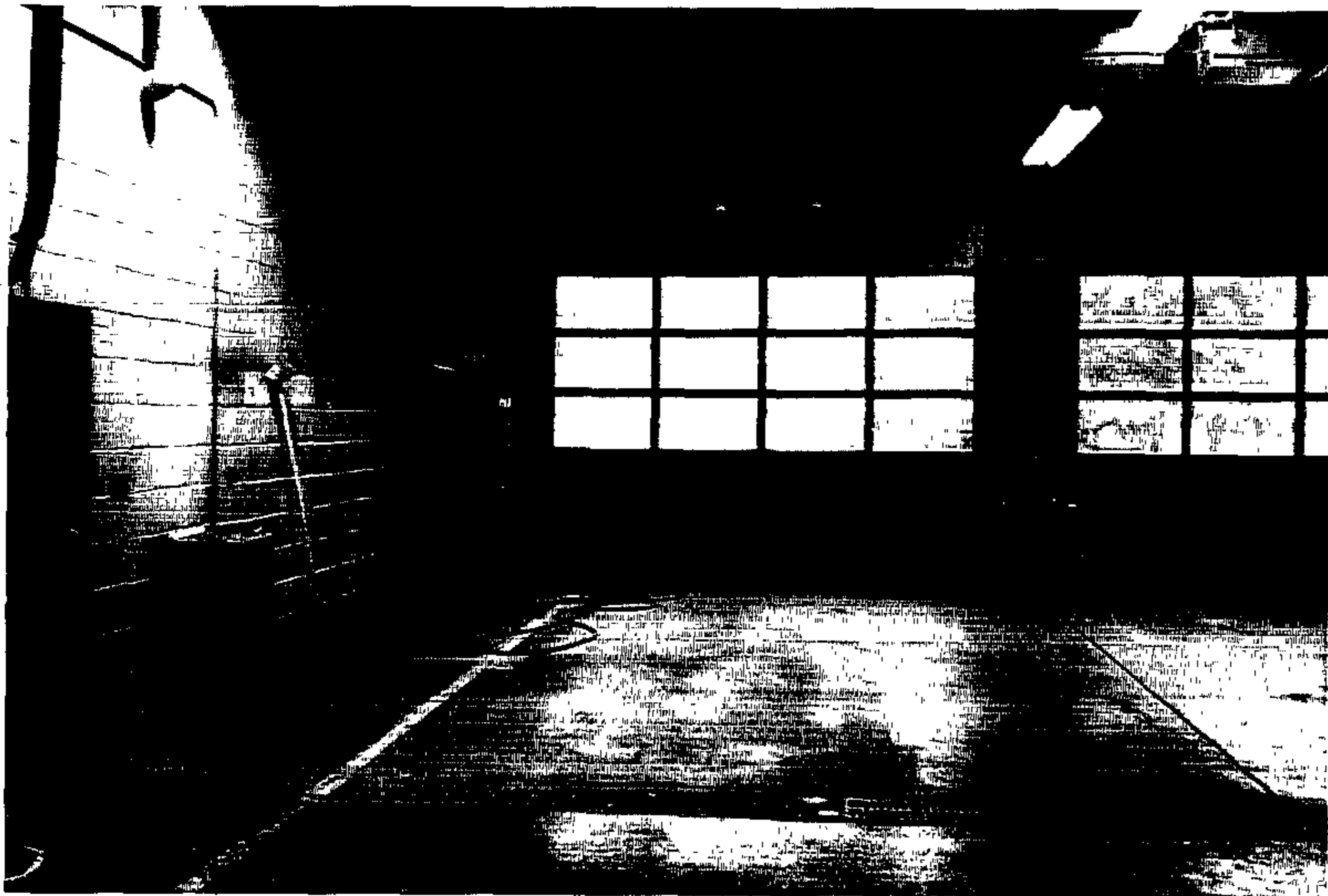
M. Interior of present building looking out toward high bay doors.
