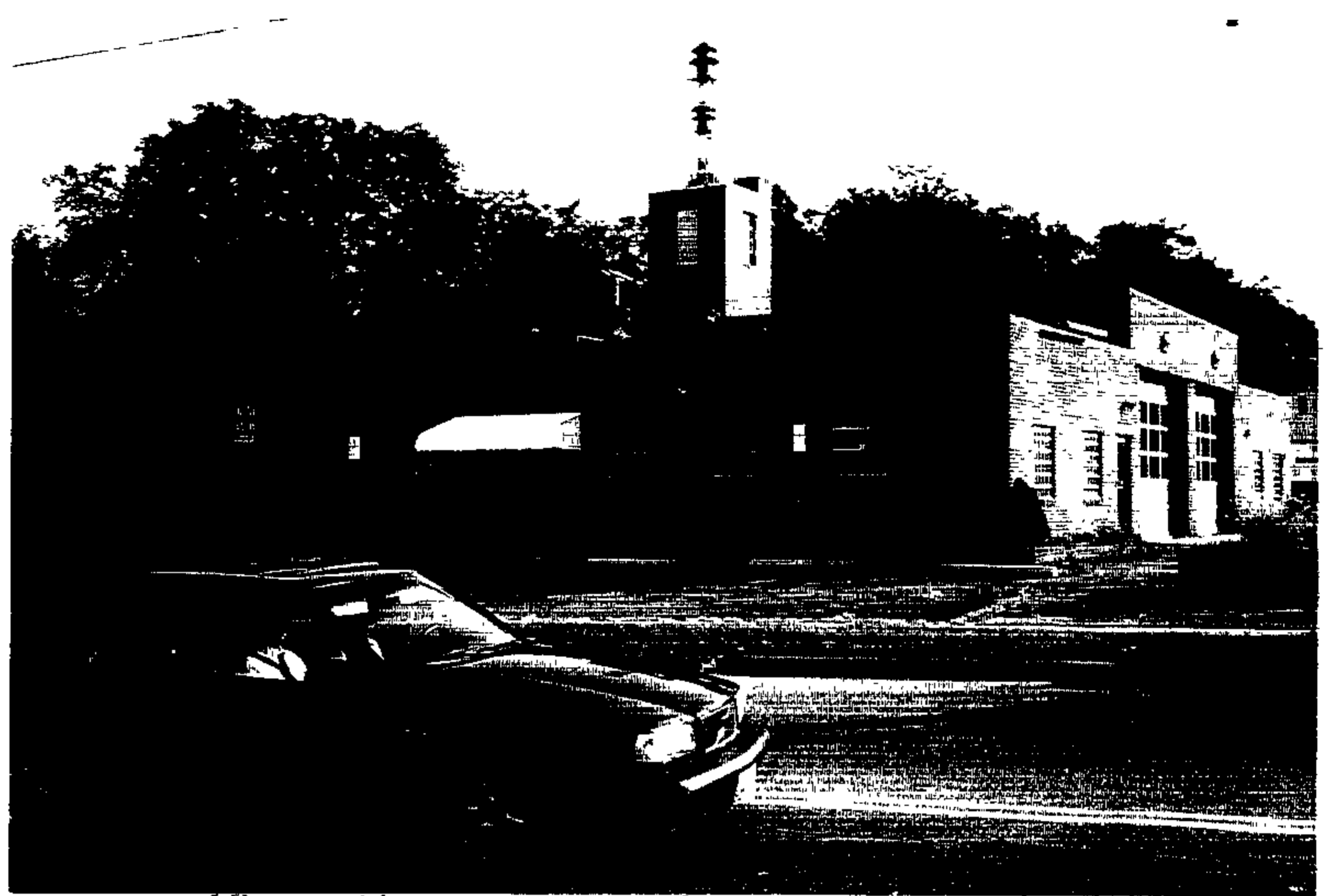
B. N/S of WVFD from corner
