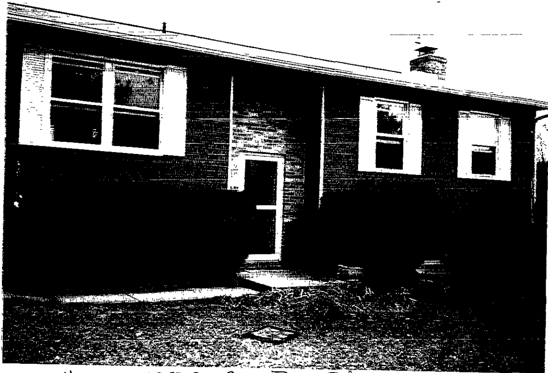
House - 19009 Grove Run Rd
