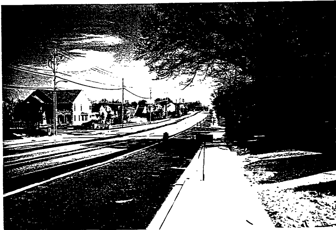
VIEW WALKING NORTH ON BELAIR ROAD APPROX 1 BLOCK SOUTH OF PROPERTY
