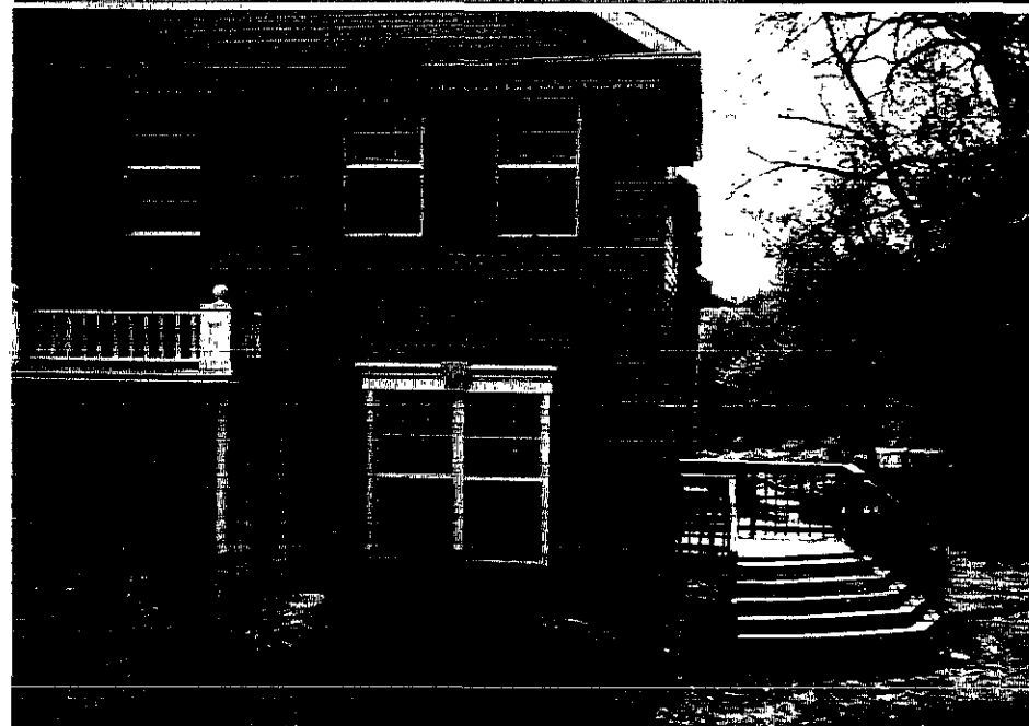
11132 HOLLOWBROOK ROAD - ADJACENT HOME - SHOWN WITH REAR DECK.
