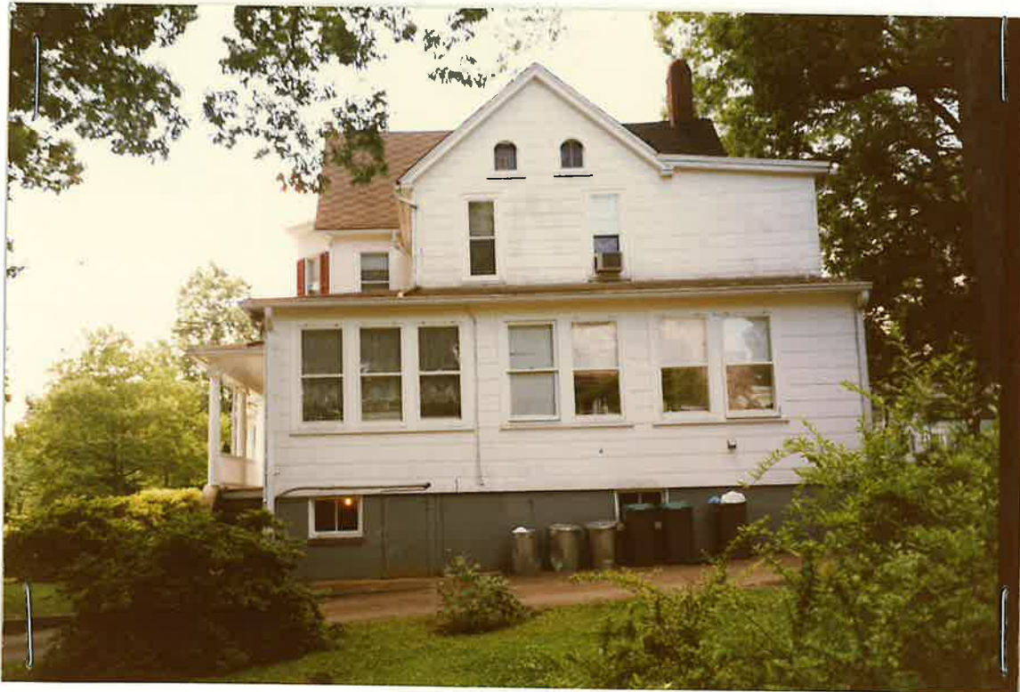
101 Beechwood Ave. - East Side
