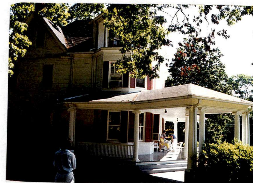
SOUTHWEST CORNER, COVERED DROP OFF.
