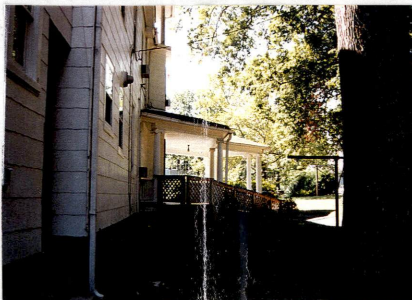
REAR PHOTO OF RAMP & SIDE PORCH. W DROP OFF
