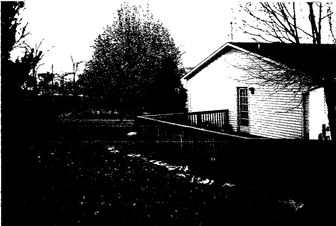
Side of Existing Home as Viewed from the Addition Side (From Rear).
