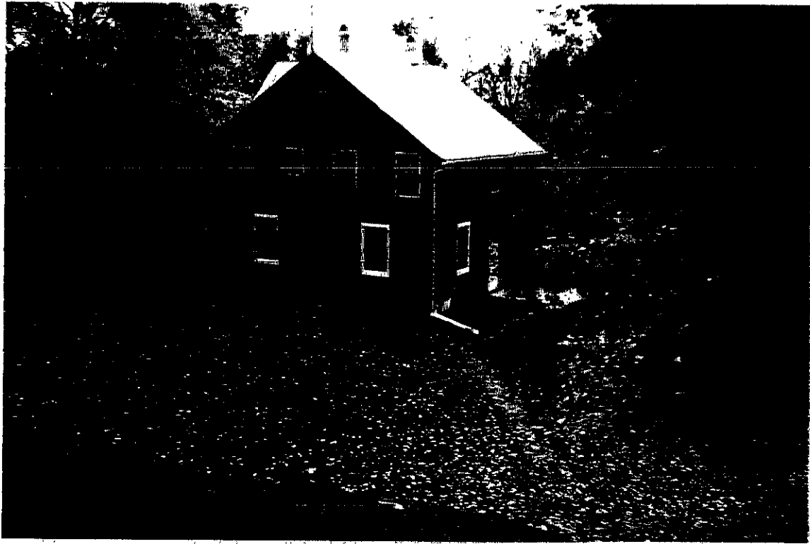
Roof view toward house
