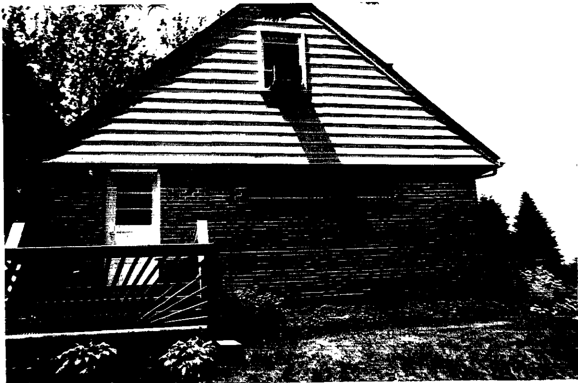
A side view of the Ledford's home. This is where the addition will be built.
