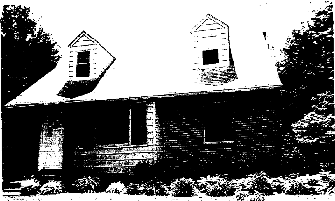
A front view of the Ledford's home. The addition will be on the left side of this photo.
