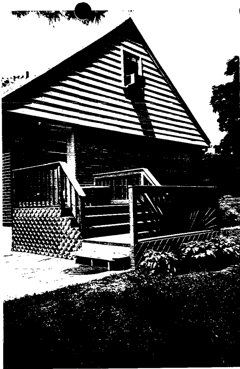
Another side view of the Ledford's home. This is where the addition will be built.
