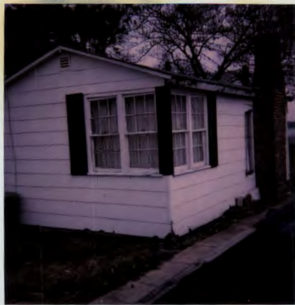
4116 BEACHWOOD ROAD STORAGE 2
