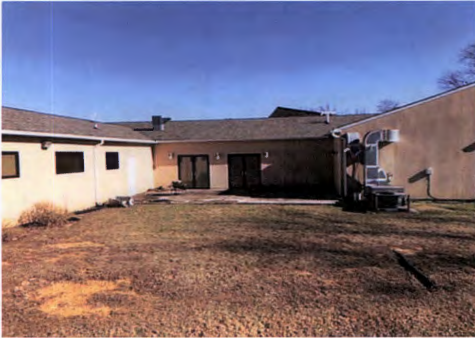
Rear (Northern) building expansion area
