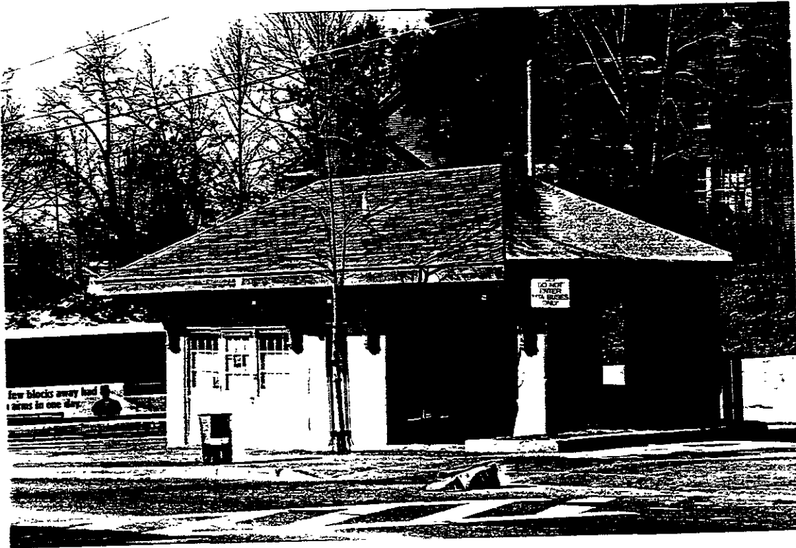
1. PERSPECTIVE VIEW OF THE FRONT OF THE BUILDING LOOKING SOUTH.
